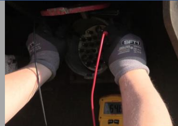
Multi-Meter used to test all 27 trainline connections
