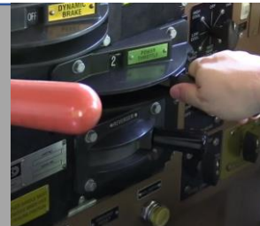
Same Electrician activates in-cab switches and controls ...
